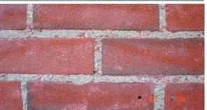
Brick or block -- it doesn't matter. Workers with pressure washers can and do damage new masonry buildings. Shown here -- wand marks on block (T), and damaged joints and wand marks on brick (B) could have been avoided with use of less pressure and more gallons per minute.
